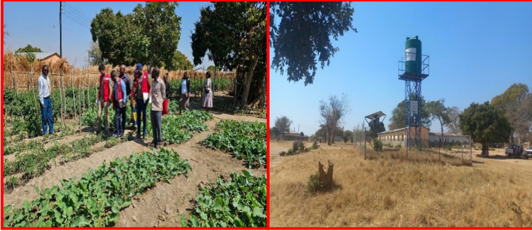
Fig 25: Solar powered reticulation systems, erected and supporting agriculture in Kapiri Mposhi
